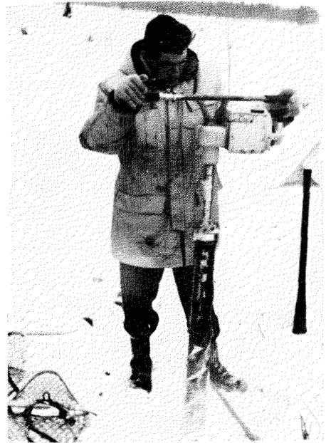
Fig.1. SIPRE ice-corer with McColloch chain-saw motor.
