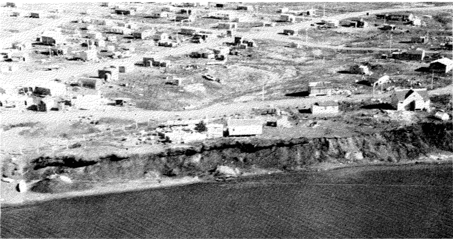
FIG. 3. Aerial view of the bluffs near the village recently settled. One building collapsed and one has been moved from the bluffs as a result of the 1968 storm. The beach formerly was 30 m. in width at this point. Photo taken in August 1969.
