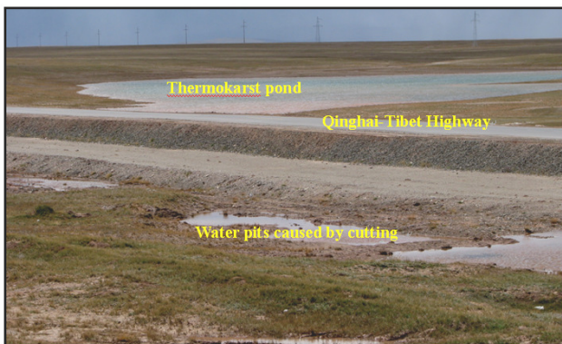
Figure 3 Thermokarst pond and small water pits developed at Chumarhe High Plateau along the QTH. These, sporadic or string-like distributed, are existed in the section of bottomland or intermountain basin with ice-saturated permafrost or massive ground-ice. The water depth is about 0.5 to 3.0 m, and the areas rang from less than 100 \text{ m}^2 to about 60,000 \text{ m}^2 .
