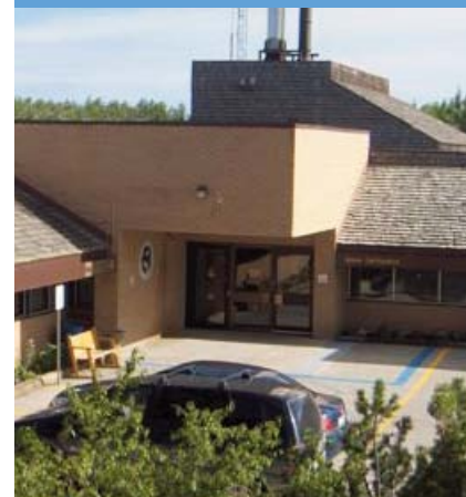
Fort Smith Health Centre
