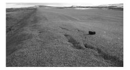
Figure 3. Thaw subsidence and cracks affecting the airfield embankment near the distance 5+230 m, Southeast side, on summer 2001 at Tasiujaq Airport, Northern Quebec, Canada. The black camera case gives the scale. (photograph by Denis Sarrazin, CEN)
