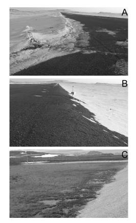
Figure 7. Snow accumulation on the Southeast (A) and Northwest (B) shoulders and toes of the airfield embankment on April 2005. C) Drainage problem at the Northwest toe of the airfield embankment on July 2004 at Tasiujaq Airport, Northern Quebec, Canada. (photographs by Frédéric Vinet, CEN)
