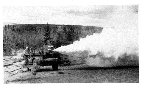
Plate 10. Aerosol generator mounted on vehicle discharging insecticide in control experiments against black flies and mosquitoes at Whitehorse.
