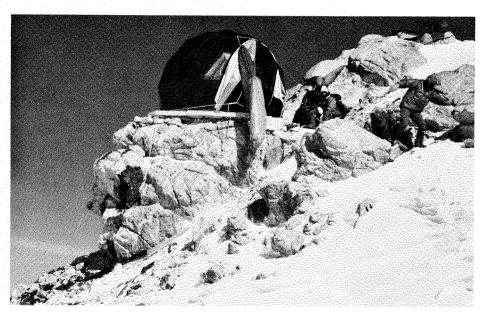
FIG. 4. Completed hut showing part of outer canopy pealed back over inner nylon cover. (G. Holdsworth).
