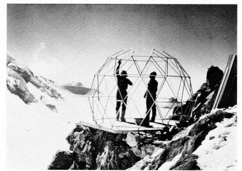
FIG. 3. Partly completed frame showing elemental structure. The NW Col is to the left. (Photo by J. Wyss).
