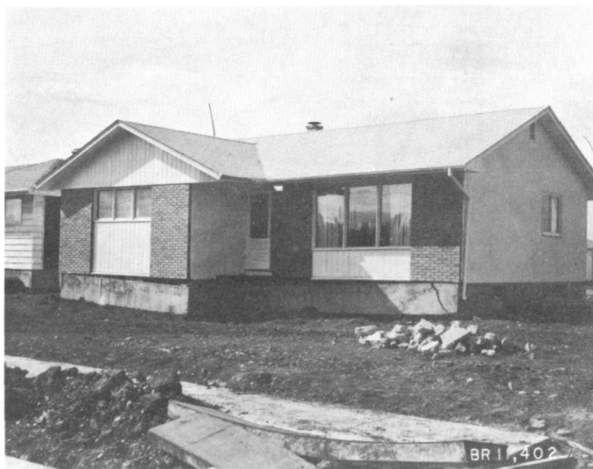
Fig. 2 Thawing of permafrost has caused house foundation to settle unevenly.
