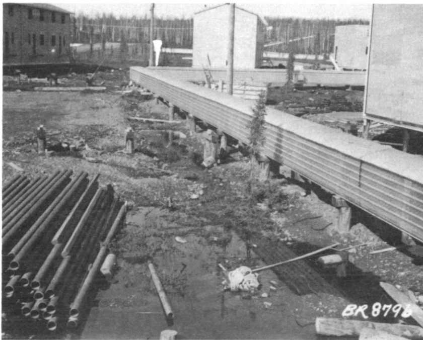
Fig. 7 Pile foundation prevents thawing of permafrost under large oil tank.
