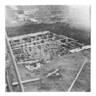
Fig. 2 Pouring first lift of boiler room piers. Note crane holding concrete hopper. August 30, 1957.
