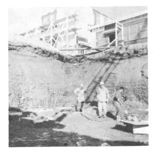
Fig. 1 View towards the northwest corner of the excavation for the boiler room piers. Note the depth of excavation - approximately 16 ft. below grade. August 29, 1957.
