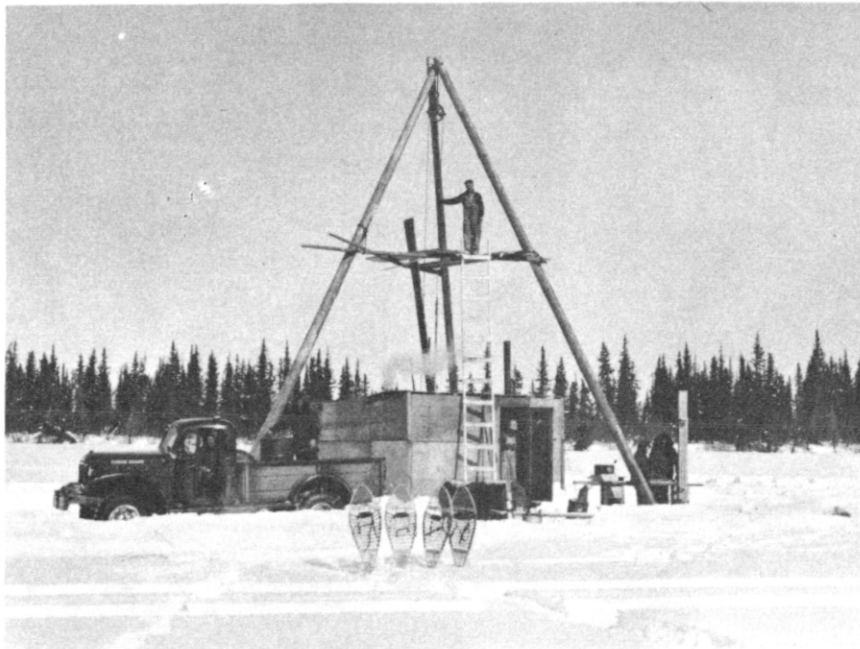
Fig. 4 Drill set-up at Hole No. 1 (centre of lake). Note core sampling table to right of drill shack and depth of snow cover.
