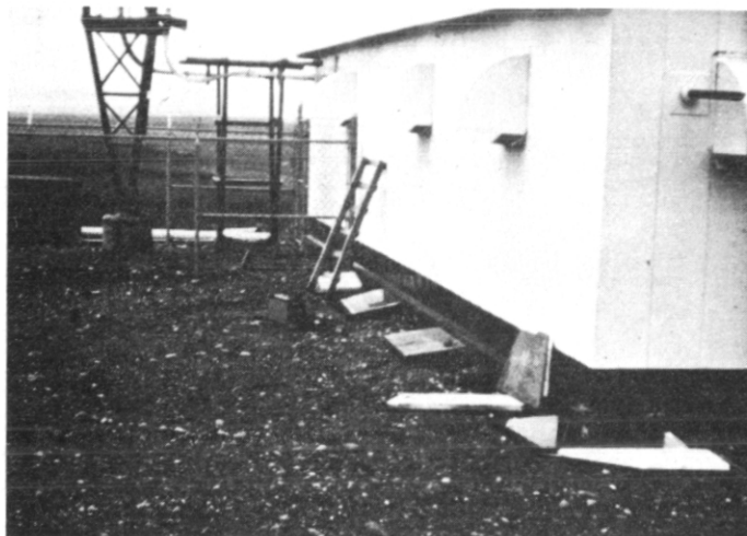
FIGURE 3 BUILDING SUBJECT TO 22 IN. OF DIFFERENTIAL SETTLEMENT DUE TO THAWING PERMAFROST
