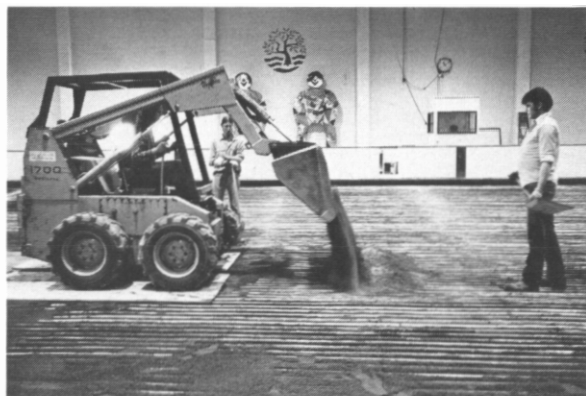
FIGURE 8. Placing sand over cooling brine pipes.
