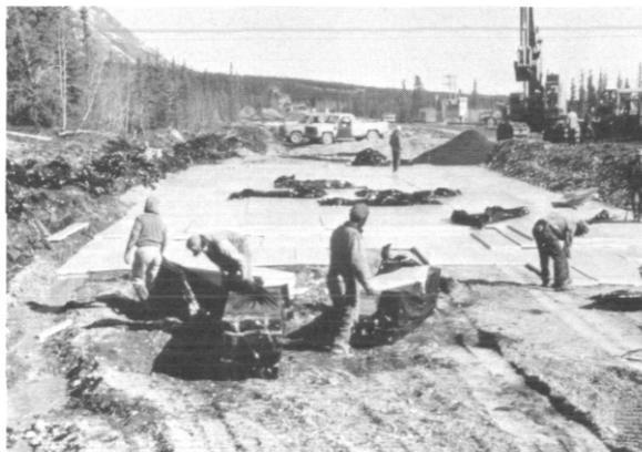
FIGURE 8. Photo showing installation of ground surface insulation.
