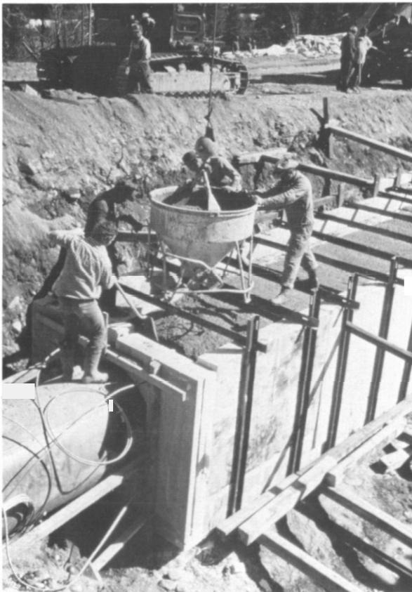
FIGURE 5. Photo showing placing of concrete inside insulation box.
