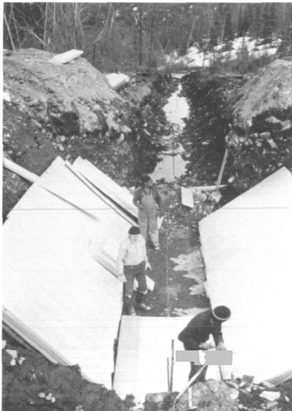
FIGURE 7. Photo showing insulation of drainage ditch.
