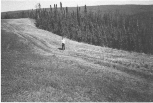
FIGURE 2. Thermokarst depression encompassing the travel lane of the workpad.
