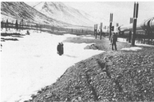
FIGURE 3. Differential settlement of the workpad in an elevated pipeline segment.
