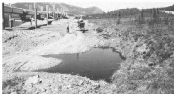
FIGURE 13. Ponding on, and adjacent to, the workpad in an elevated pipeline segment.
