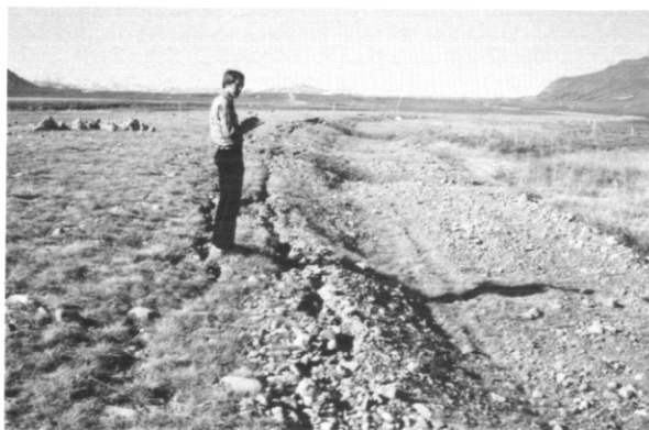
FIGURE 7. Cracking adjacent to a buried pipeline with mounding over pipe centreline.
