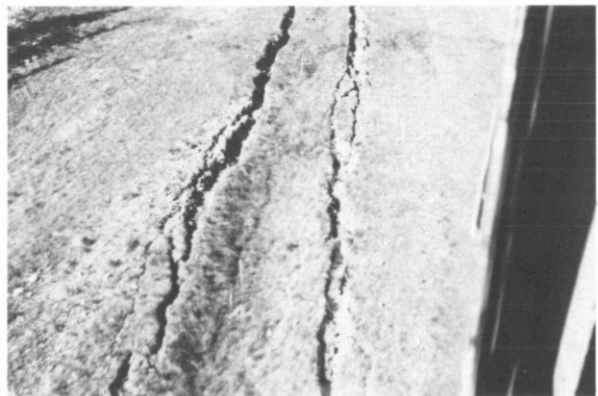
FIGURE 5. Cracking adjacent to a buried pipeline with a depressed area over pipe centerline.
