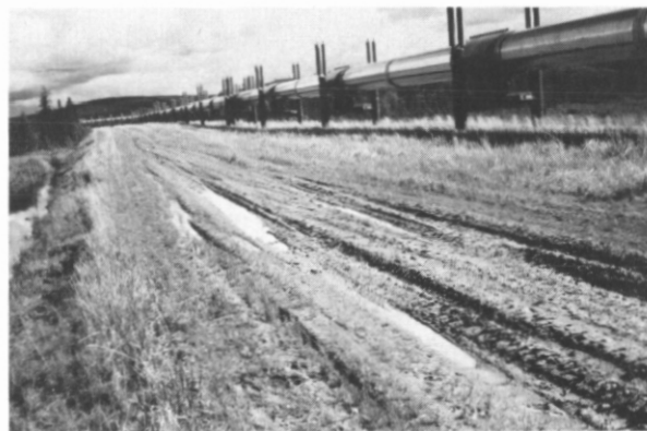
FIGURE 14. Soft, saturated, and badly rutted workpad.
