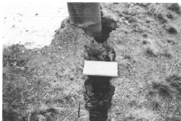
FIGURE 8. Lateral workpad movement on a cross slope with resulting mounding on the uphill side of the vertical support member and a gap on the downhill side.
