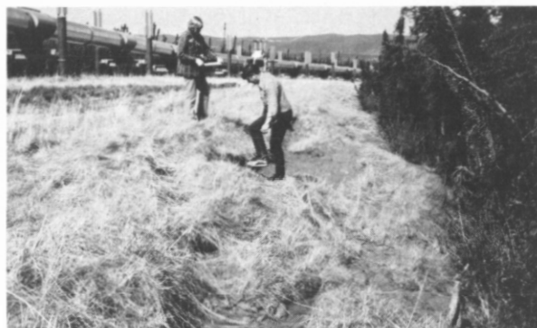
FIGURE 12. Edge of workpad mudflow failures. Saturated fine-grained workpad material.
