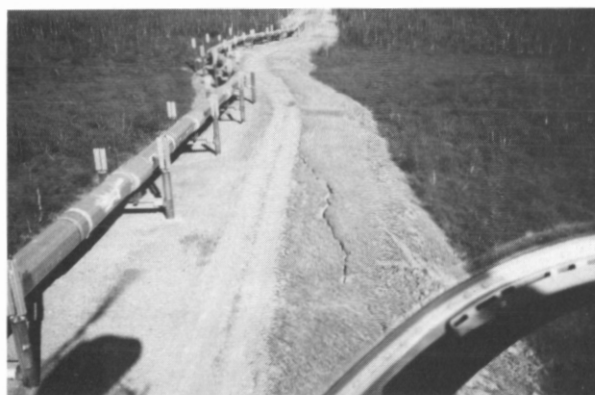
FIGURE 11. Longitudinal tension cracks on the workpad in an elevated segment of the pipeline.
