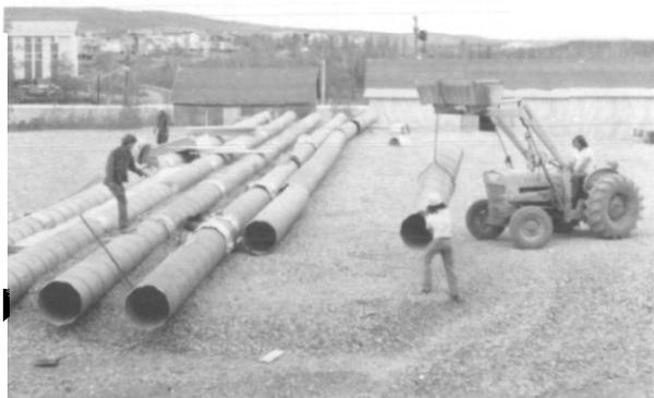
FIGURE 9. Placing and aligning ventilation culverts in granular pad.
