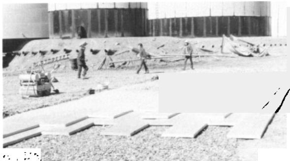
FIGURE 6. Placing the lower layer of styrofoam HI-60 insulation on the basal levelling course.
