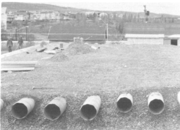
FIGURE 10. Completed installation of ventilation culverts in the granular pad.
