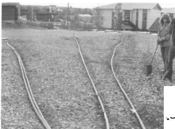
FIGURE 12. Thermistor leads carried through the fill in plastic conduits.
