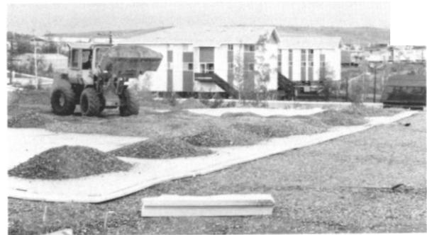
FIGURE 8. Placing crushed dolomite on the upper insulation layer.
