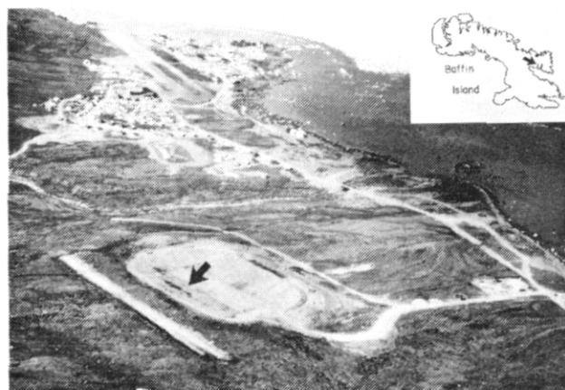
Figure 1. View of the new reservoir at Pangnirtung reservoir (in the foreground) during construction in July 1987 showing relation to Duval River and Pangnirtung Fiord (at arrow on inset map). Ice wedges observed in 1986 were exposed at the arrow on the photograph.
