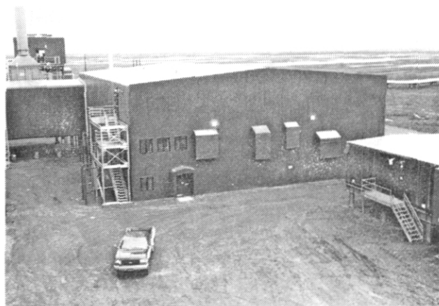
Figure 4. Cpf-3 work area/office building (thermosyphons are not visible).
