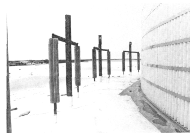
Figure 5. Divert tank with thermosyphons and supports shown.
