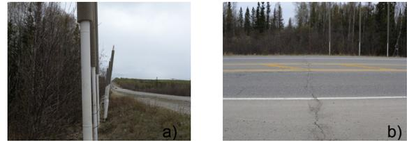
Figure 9 a) Evidence of settlement and frost jacking of thermosyphons and b) contraction crack in the pavement.
