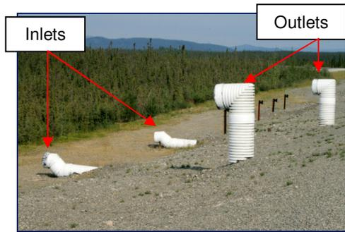
Figure 11 : Inlets and outlets of the longitudinal culvert system (section 7).
