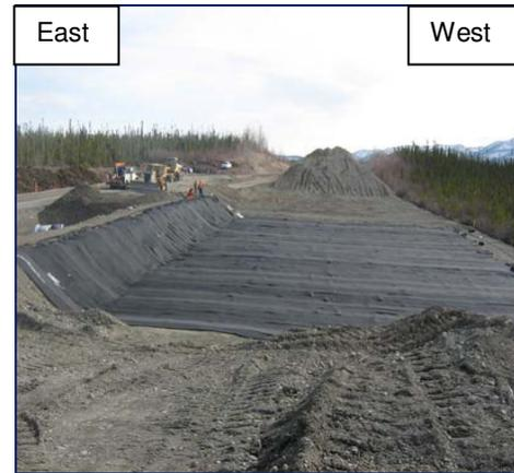
Figure 7: Placement of the heat drain across the full width of the embankment (section 2)
