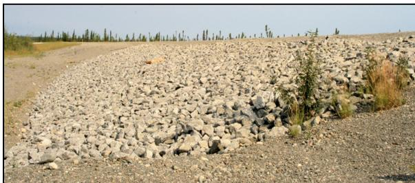
Figure 4 : Air convection embankment uncovered
