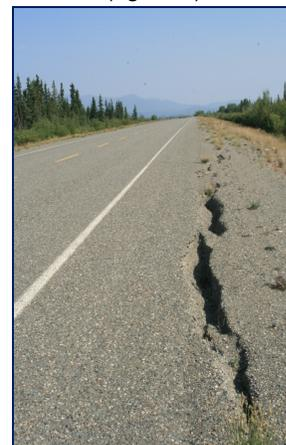
Figure 1 : Longitudinal cracking observed along Alaska Highway (2009)
