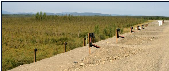
Figure 9: Heat drains on side slopes (section 4)
