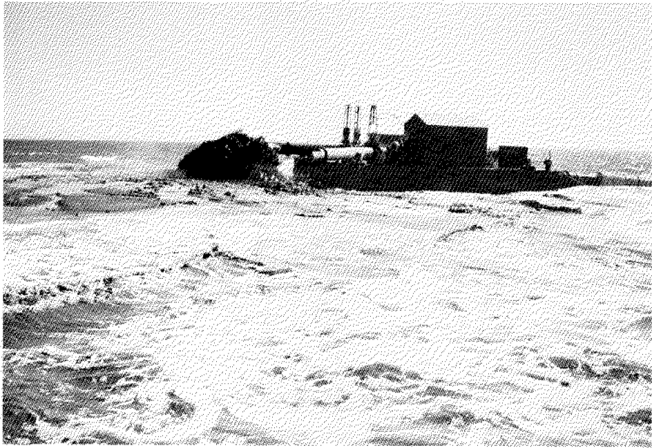
Plate I Shore pontoon with suction dredge discharging onto the surface of Isserk F-27, July 28, 1977
