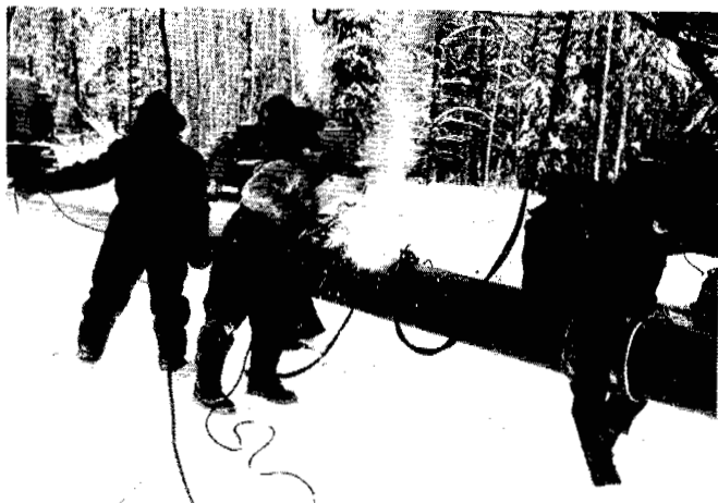
Welding together two sections of pipe.
