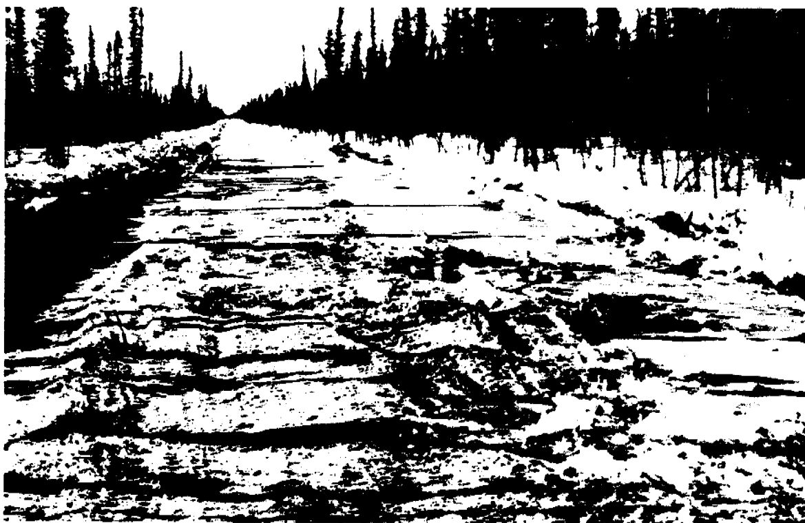
Old seismic line used as a perennial winter trail. Icings are caused by groundwater flow across road. (K.M. Adam)
