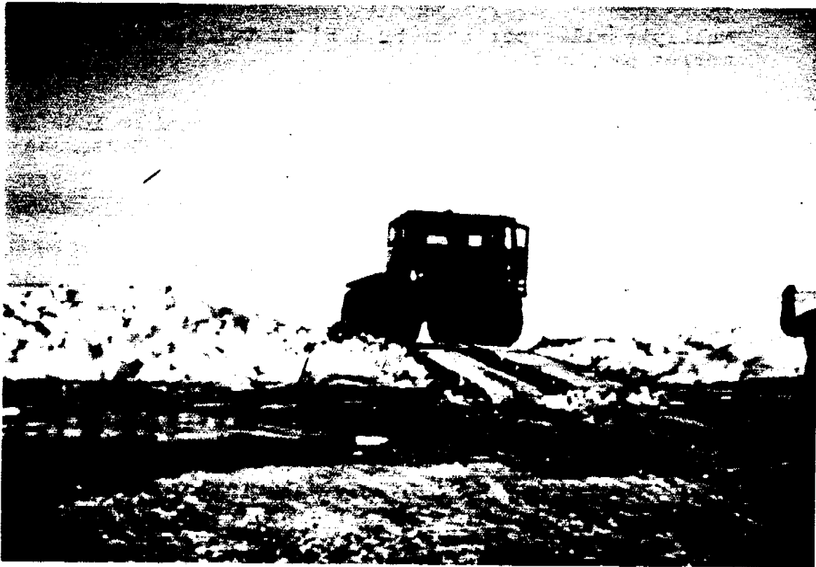
Timber ramps allow traffic to cross a pressure ridge in safety. (Department of Northern Saskatchewan)
