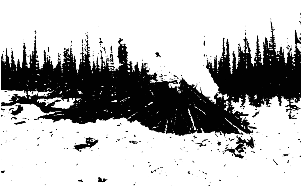
Burn piles are unacceptable in permafrost areas because they destroy the vegetative mat. (K.M. Adam)
