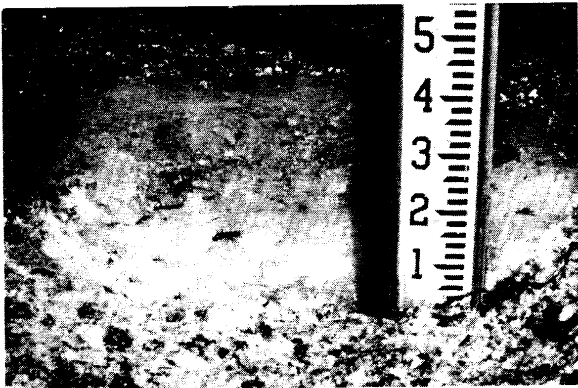
Cross-section of a solid ice road. The ground was covered with a layer of snow before watering started. (K.M. Adam)
