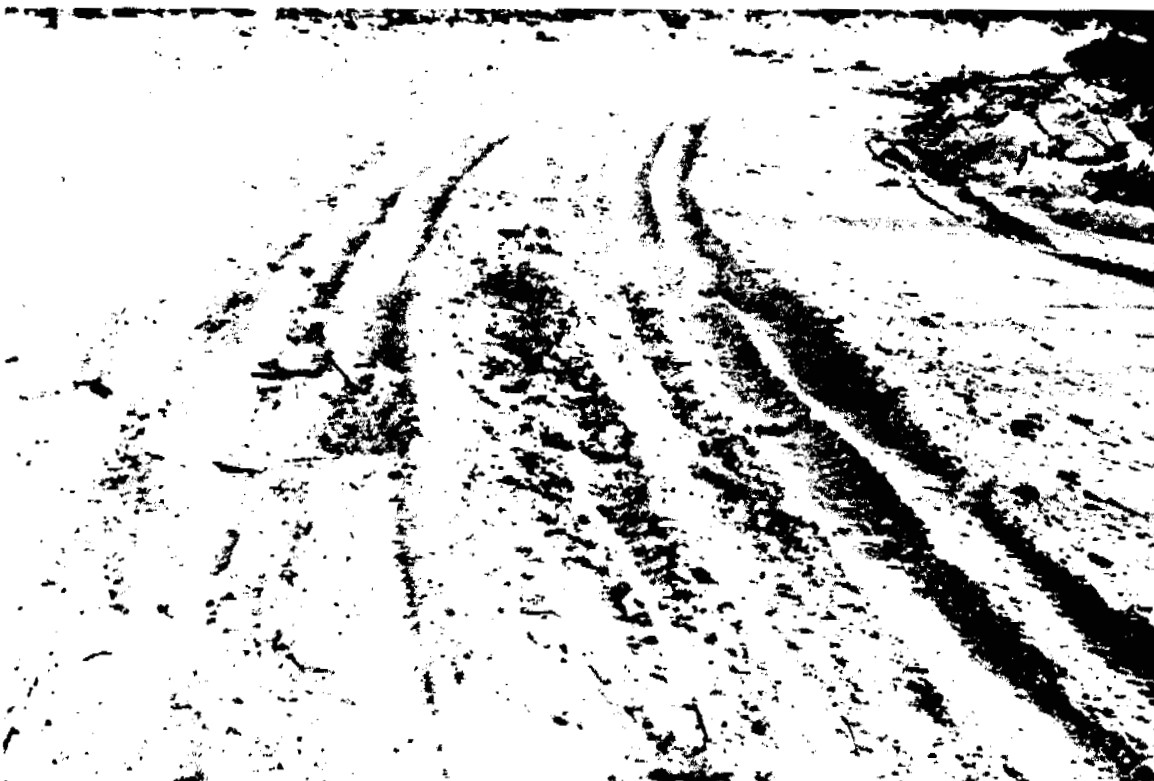
Rutting of an insufficiently compacted snow road after fewer than 20 passes of a light van. (K.M. Adam)
