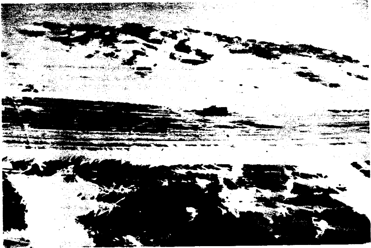
Winter road on ice. Cracks are caused by changes in temperature. (Department of Northern Saskatchewan)
