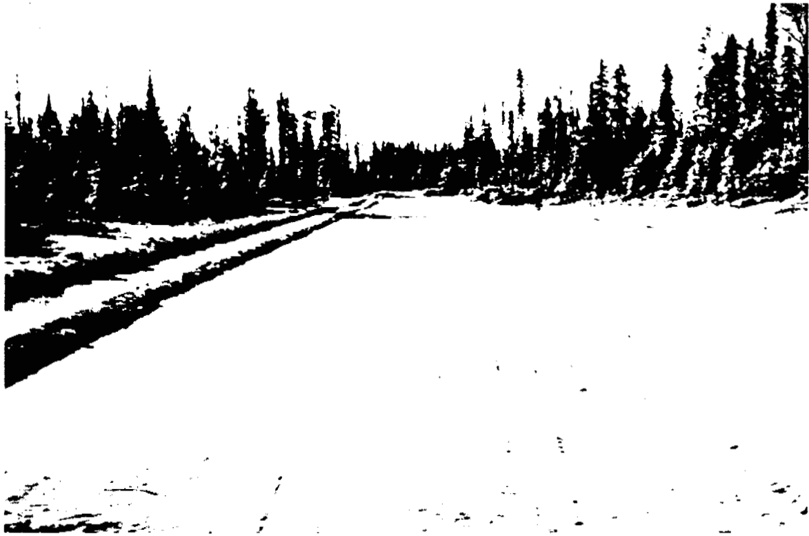
Ice-capped snow road in northern Ontario used for hauling logs. Lane on left is ice-capped for loaded vehicles. Other lane is compacted snow for the return trip.
