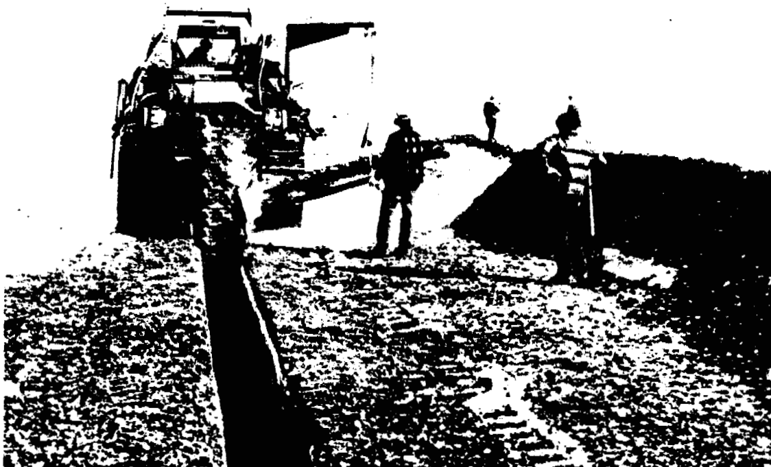
Building the Alyeska gas feeder lines through a snow work pad. Note 48-inch Alyeska oil pipeline in background at right. (Joint Fish and Wildlife Advisory Team)
