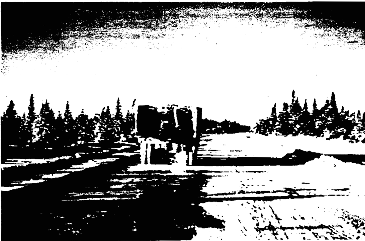
Flooding the haul lane of an ice road used for transporting logs.
