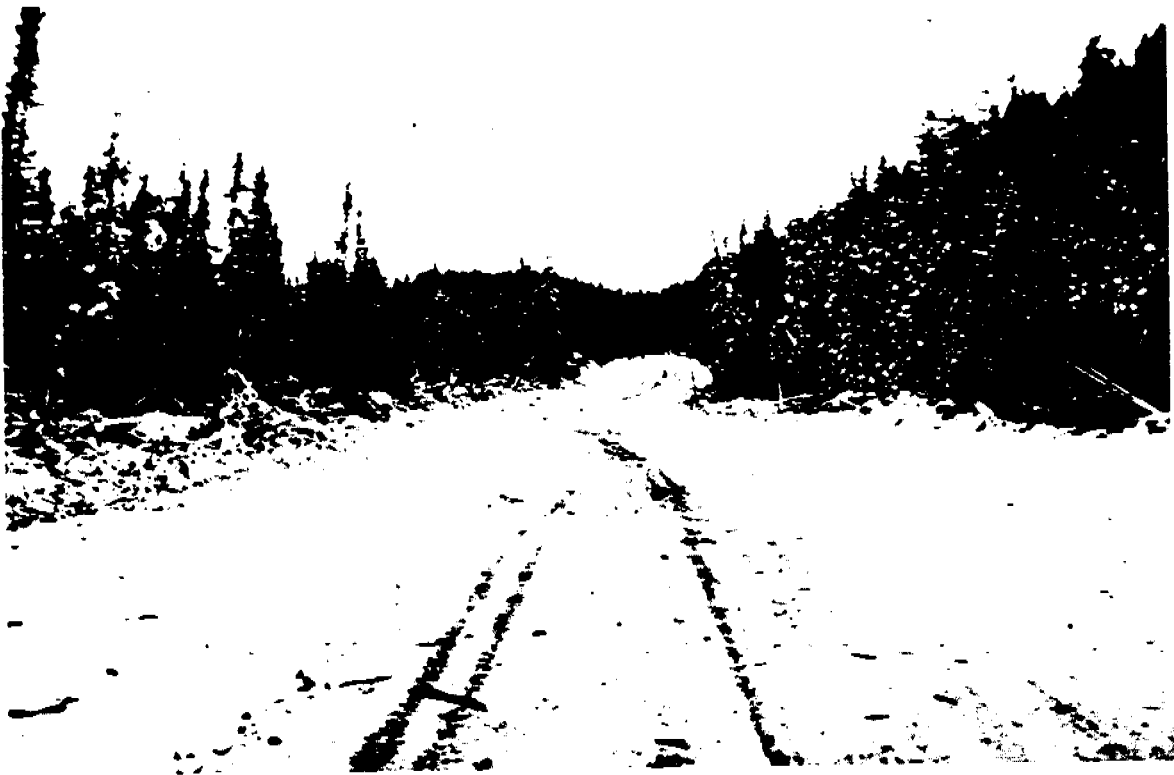
Temporary trail through a nonpermafrost area. Note mineral soil on the road and slash windrowed along left-hand side. (J.D. McMillan)
