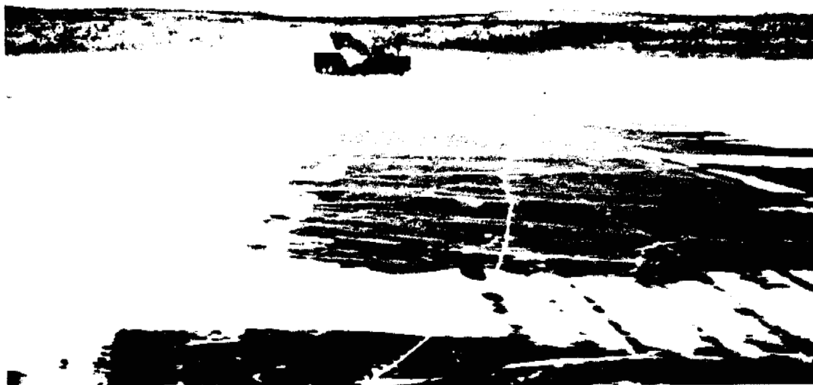
Snow from surface of lake to be used to build a compacted snow road. (K.M. Adam)
