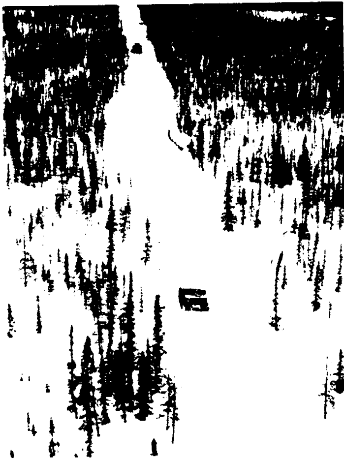
Temporary trail through a nonpermafrost area. Note mineral soil on the road and slash windrowed along left-hand side. (J.D. McMillan)
