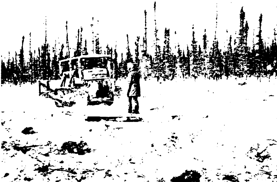
Steel drags achieve a smooth roadway but tend to scuff the surface. (K.M. Adam)
