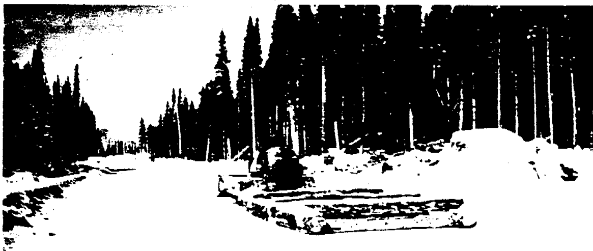
Large-diameter roller for compacting snow. The device on the front of the tractor is a makeshift snow processor. (K.M. Adam)
