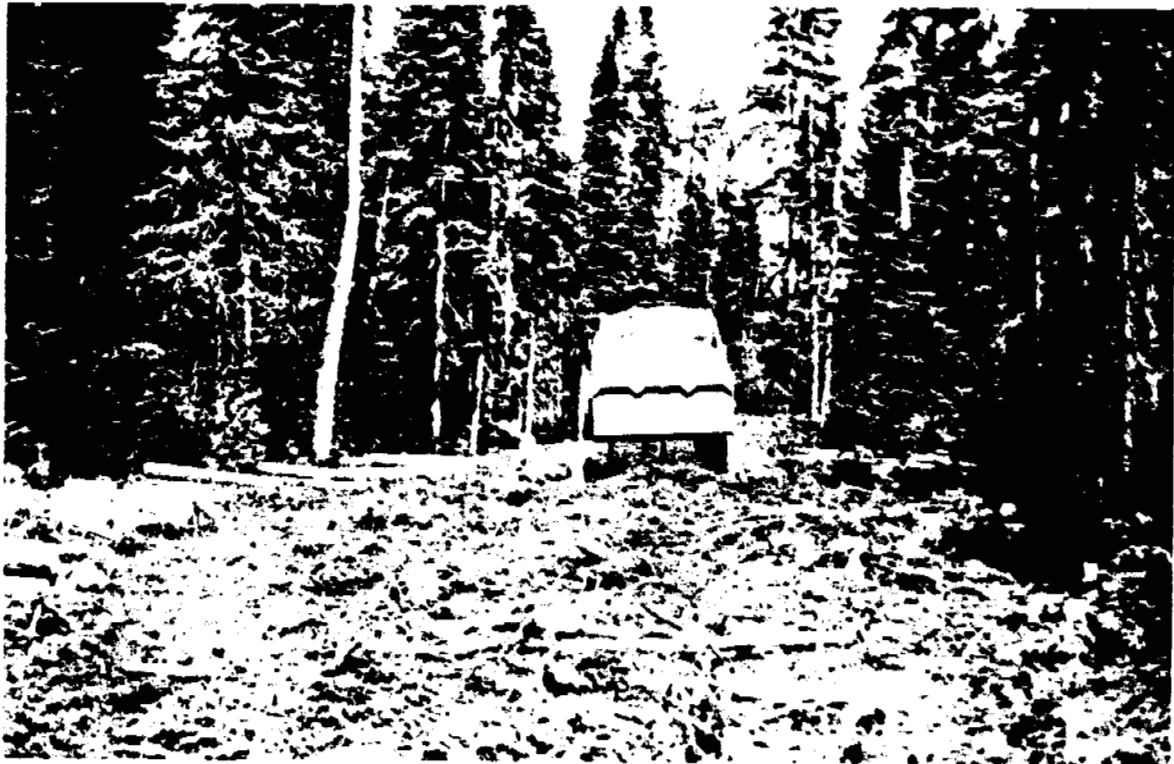
Granular material being used to fill holes on a right-of-way. The practice is typical in nonpermafrost areas.
