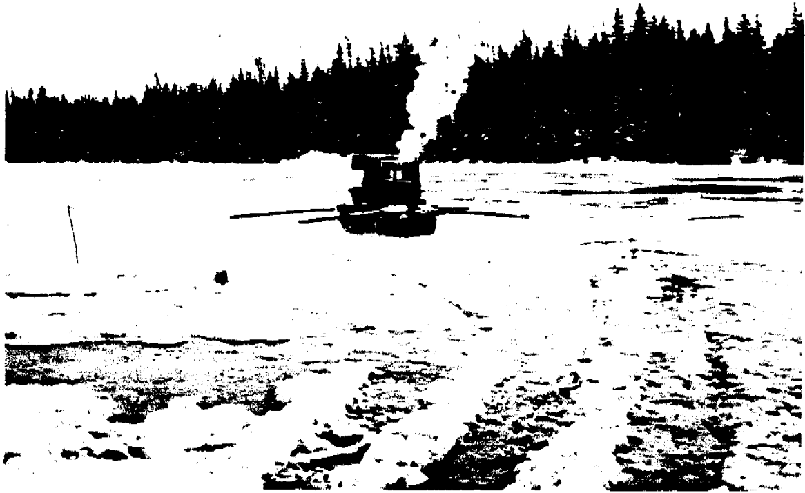
A J-5 compacting slush to speed thickening of the bridge.
