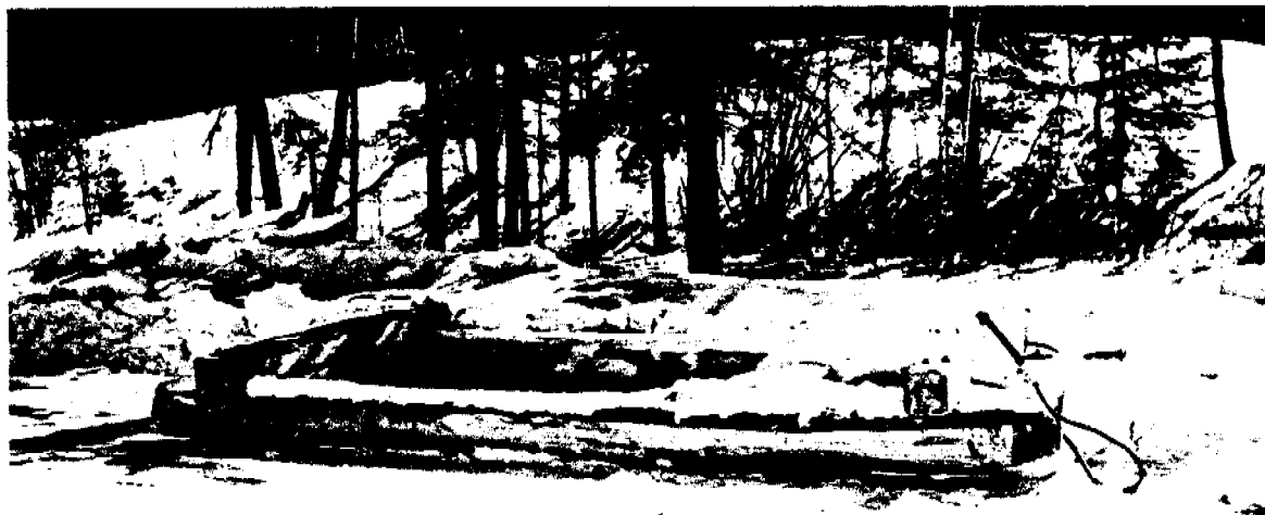
Steel drags achieve a smooth roadway but tend to scuff the surface. (K.M. Adam)
