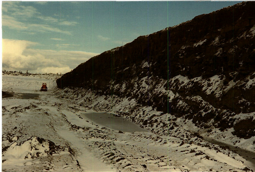
Photo No. 1 Source 500 showing existing pit wall exposure.
