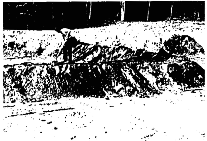
Class 4 material used as a berm around a fuel storage site
