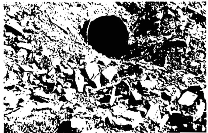
Class 5 material used as rip rap to protect a culvert outlet
