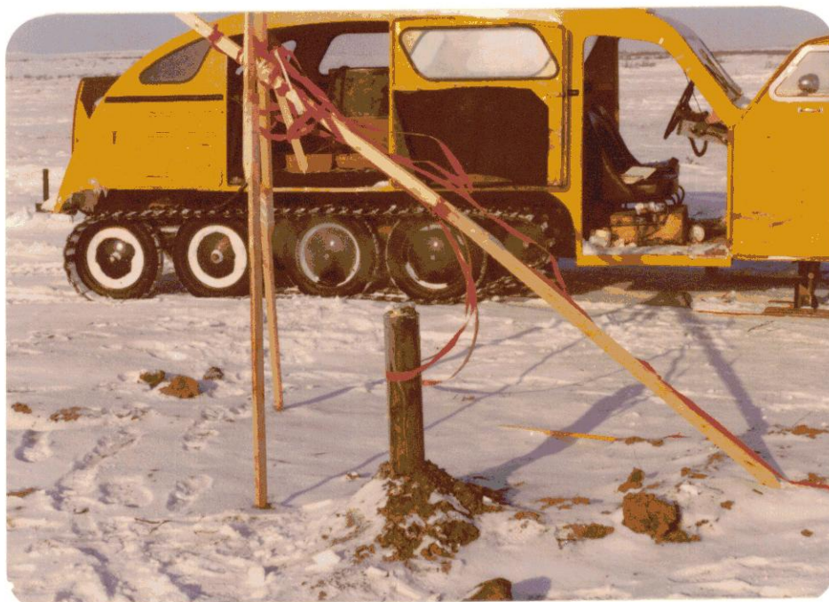
PHOTOGRAPH No. 4 Benchmark Installation.
