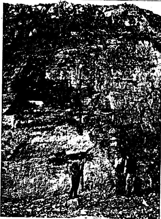
#16 Blasted Wall - thin-thick bedded, fractured, limestone (some fracturing may be blast induced)
