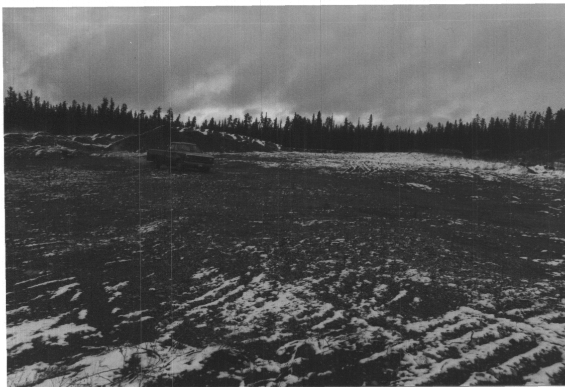
PHOTO 1: Foxhole South (Bertons') Pit Deposit 5-69. View to northeast along axis of pit, showing stockpiles of sandy gravel on left and windrows of restoration materials on right.
