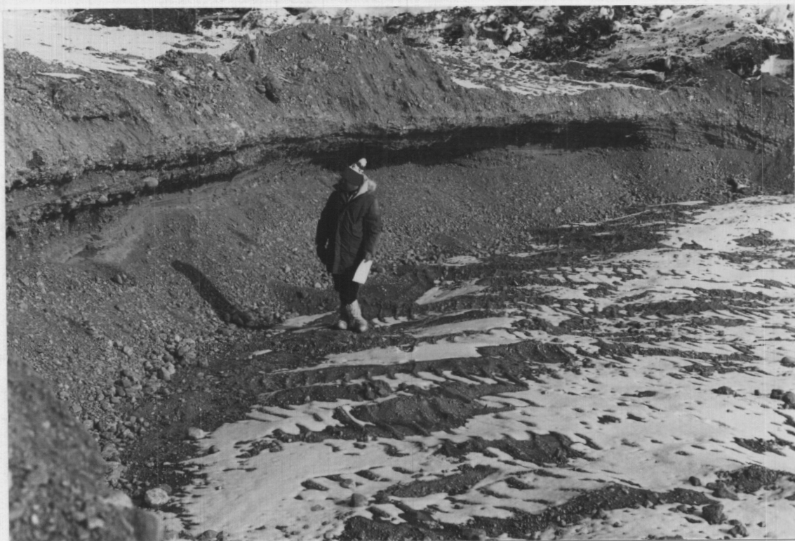
15. Deposit 5-6 (HR-109A): Small pit developed, adjacent to Fort Smith winter road alignment, by J. Pope of Hay River in well graded Class 1 or 2 aggregate.
