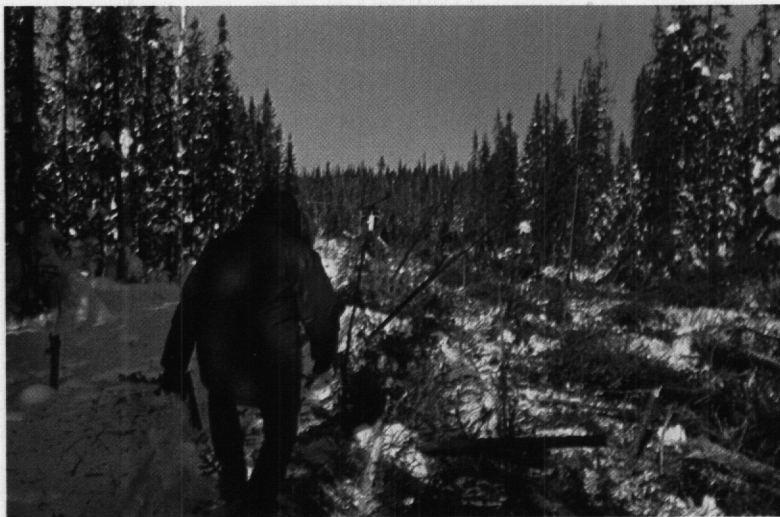
Photo 9: Start of centreline clearing - Mile 347.
