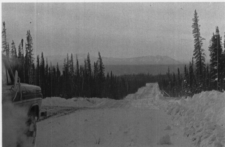
Photo 10: Highway on CNT centreline - Mile 405.
