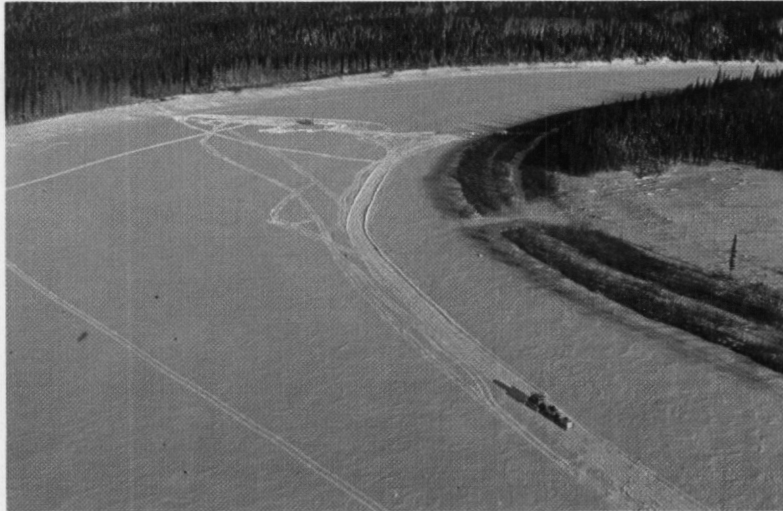
Photo 25: Drilling on ice, Willow Lake river crossing - Mile 394.
