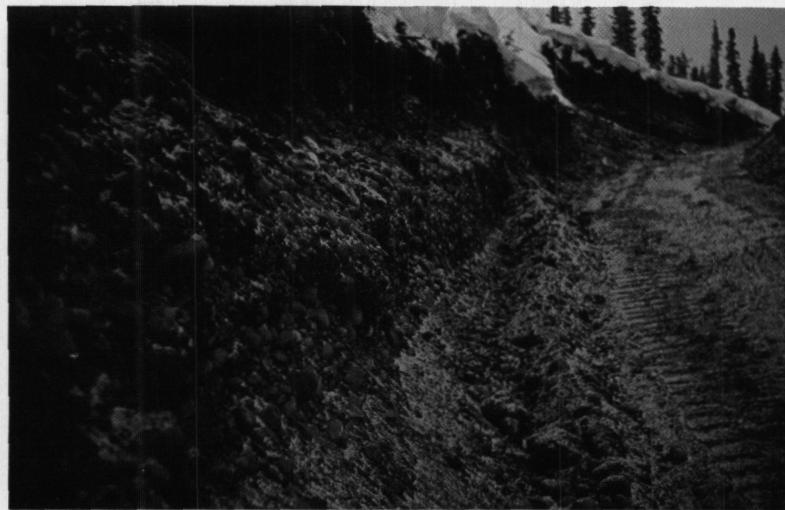
Photo 12: Gravel in trench on centreline, north bank of Smith Creek - Mile 430.
