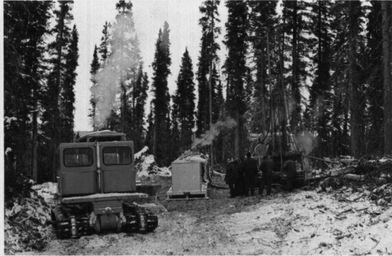
Photo 29: Drilling with mud - 80' hole in dry sand - edge of terrace - Mile 393.
