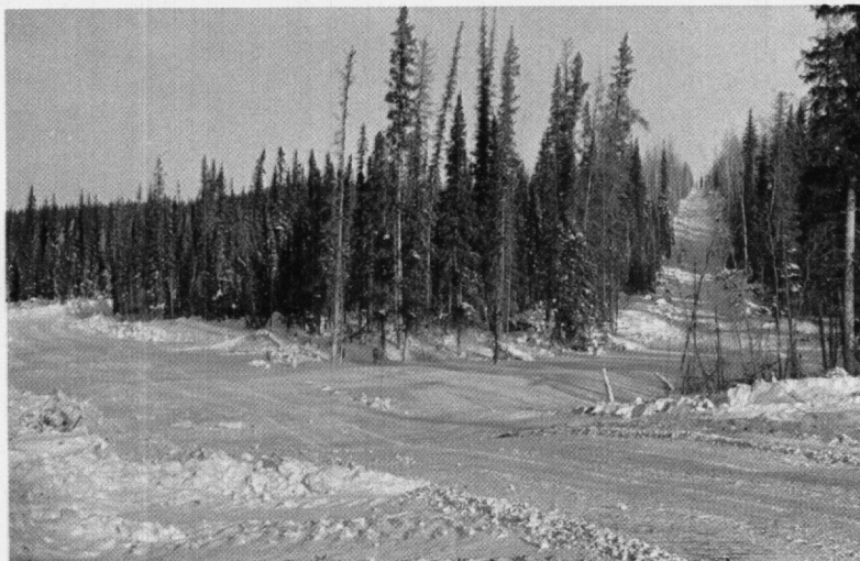
Photo 8: Icing at Mile 412.
