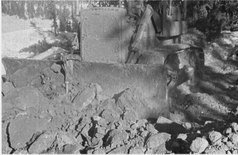
Photo 13: D-7 trenching test pit - 355-BT-1.
