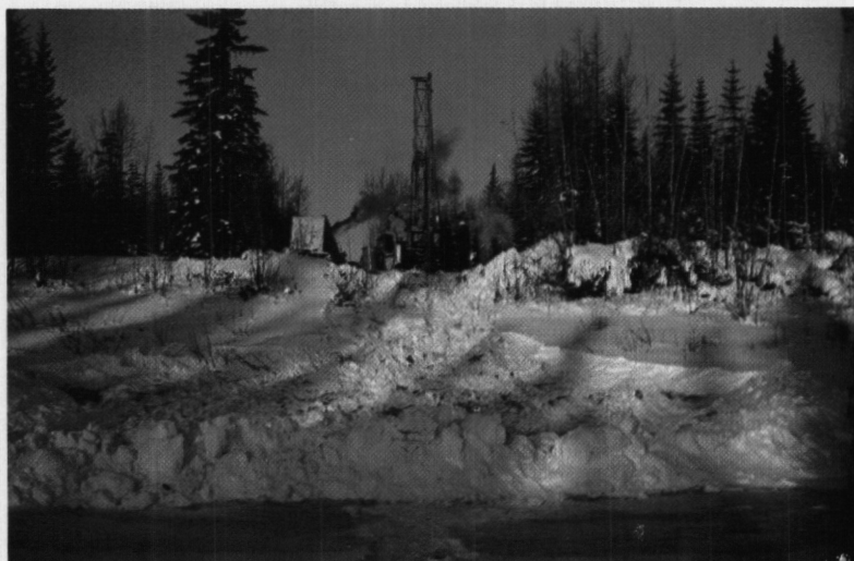
Photo 26: Drilling - north bank of River Between Two Mountains - Mile 411.
