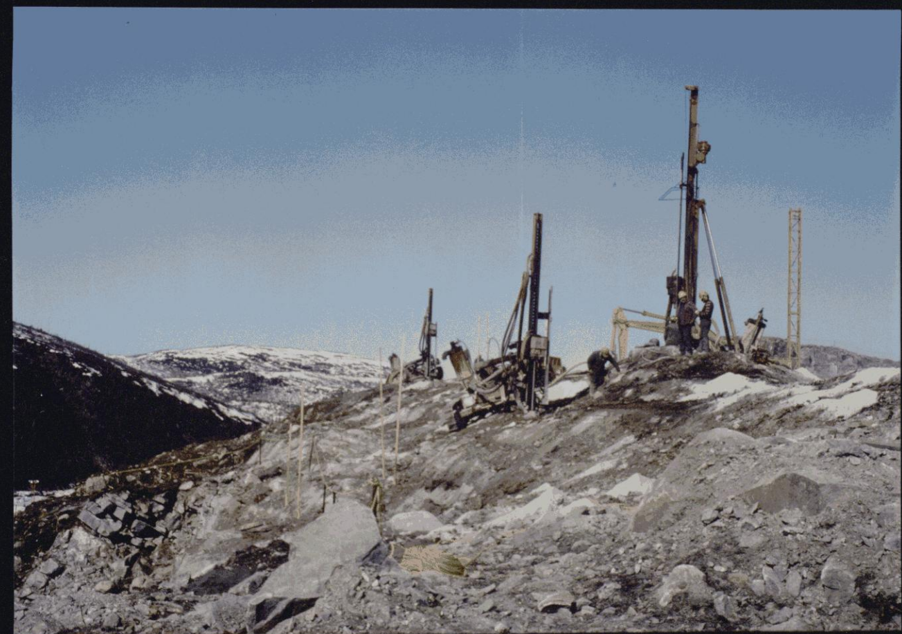
Photo 2 - Airtrack Drilling
