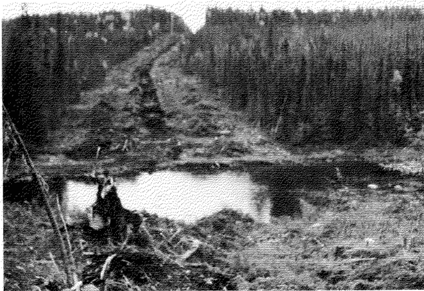
16.9.72. East bank of the Martin River. Vegetation is mainly black spruce with some aspen on peaty gleysol soils. Landform is an abandoned alluvial terrace mantled by silt and sand which is overlain by organic material. The upper 10 feet is believed to contain abundant ground ice, this is partly manifested by pools of water along R.O.W. as shown in photo.
