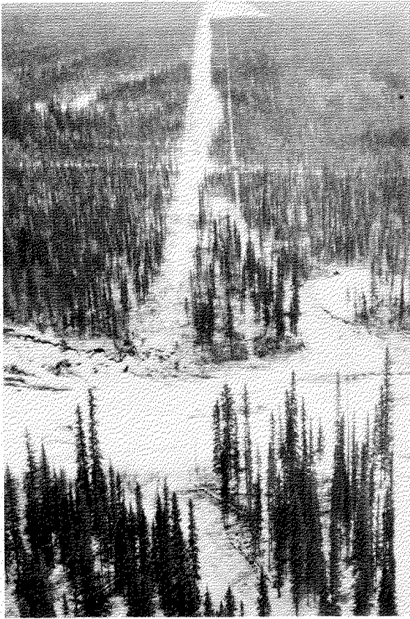
29.10.72. Little Smith Creek looking south. This approach crosses a steep glaciofluvial terrace. Stream banks appear to be easily erodible. Two span bridge more suitable for free passage of debris.
