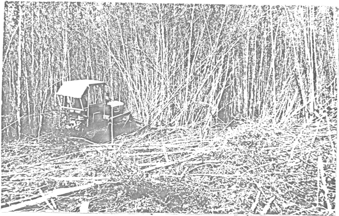
Figure 4.2 Clearing the Slave soil of light aspen tree cover using the small crawler tractor.
