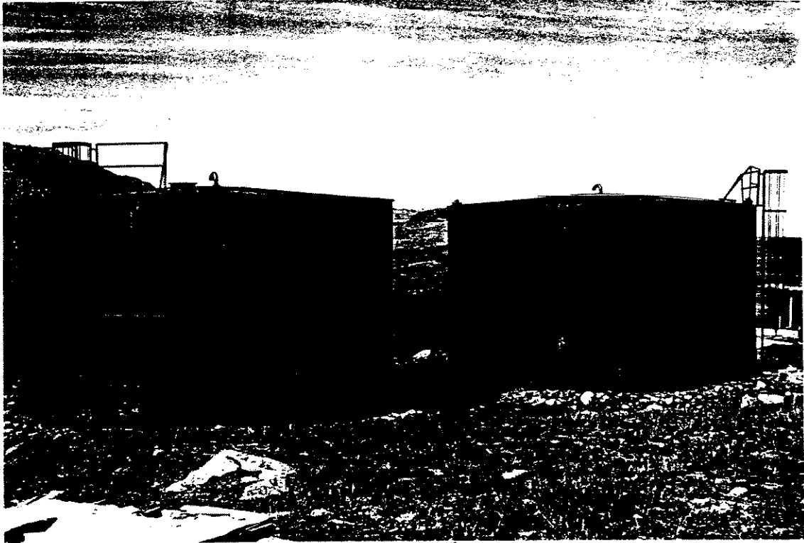
Large Fuel Tanks
