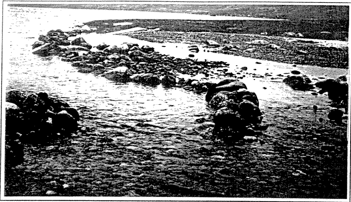
Figure 42. Paakittuq ( after remedial works): a deflection wall built at the entrance to the lake (outflow) reduces water lost through a secondary channel.
