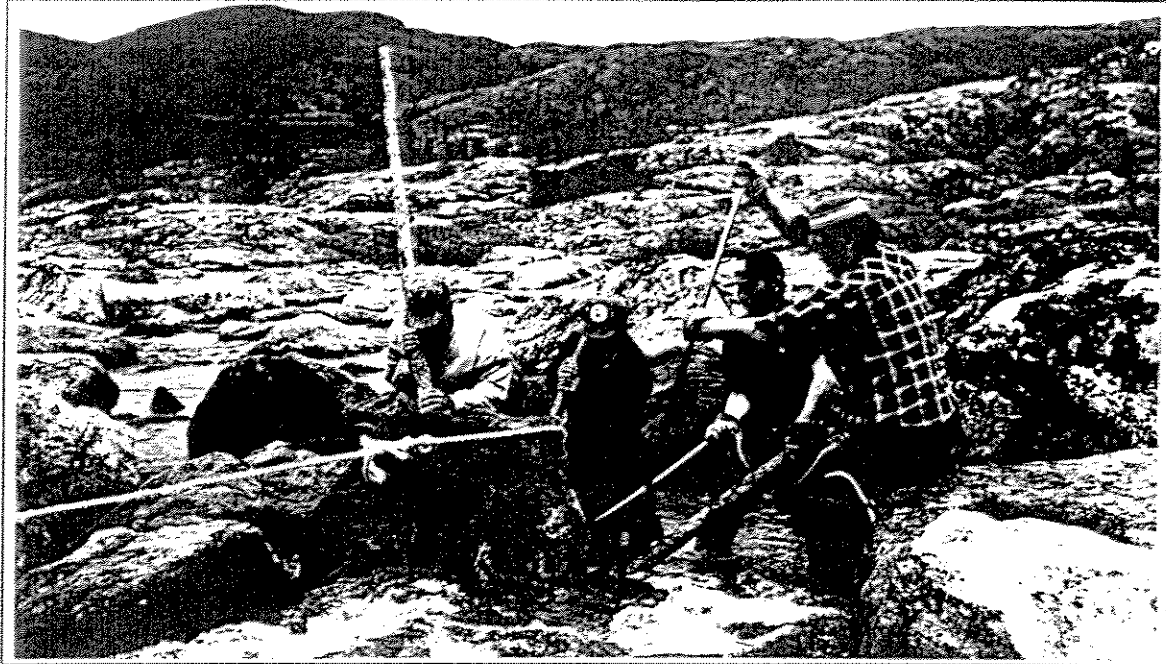
Figure 2. In Tasikallak, fishway enhancement implied moving large boulders.
