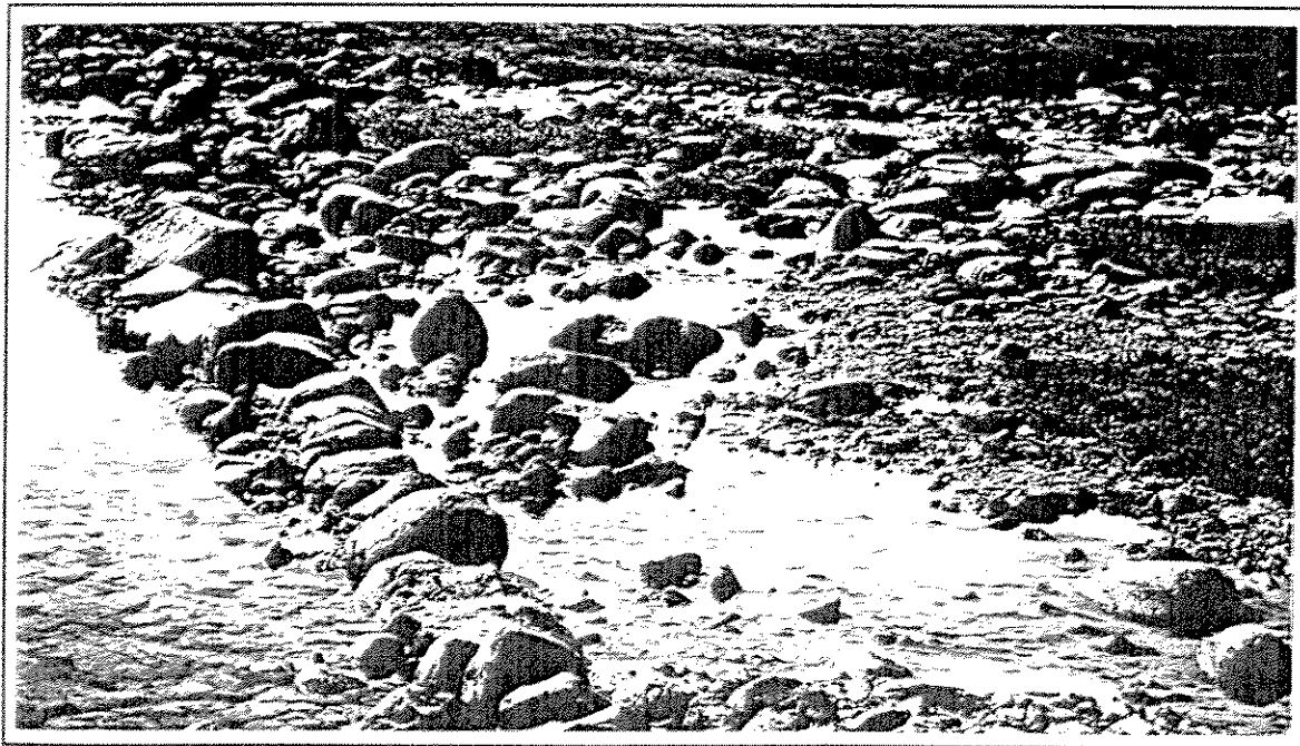
Figure 49. [View with Figure 48]. Side view of the stream just above the boulder field, showing how the deflection wall diverted the flow into the main channel.
