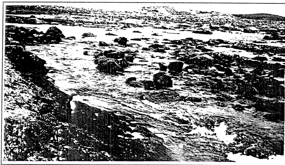
Figure 35. Although the need was questionable, remedial works were conducted in the situation illustrated above by moving rocks onto the right side of the channel. The top photograph was taken before the remedial works. The bottom photograph shows the channel immediately after the remedial works. In spite of a deflection wall (upper left corner) which partially retain the flow, the water level in the pool had already dropped by about 10 cm.
