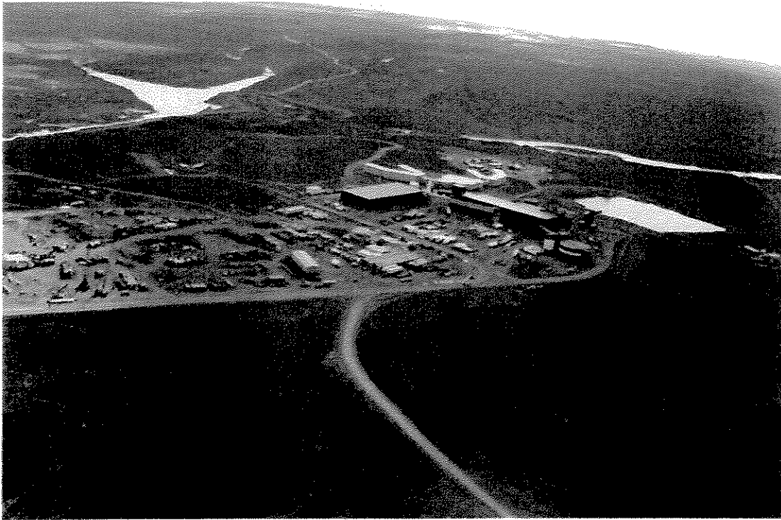
Photograph 1. Katinniq mining complex located near the confluence of the west, east, and south branches of the Deception River.
