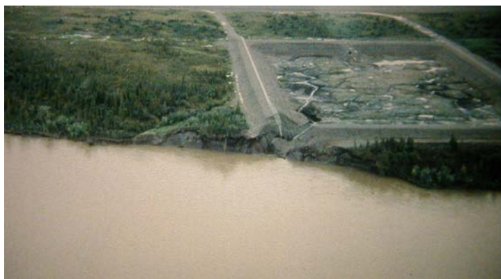
Figure 3. Permafrost thaw in concert with river bank erosion compromises a sewage lagoon. Photo by Dan Schubert.
