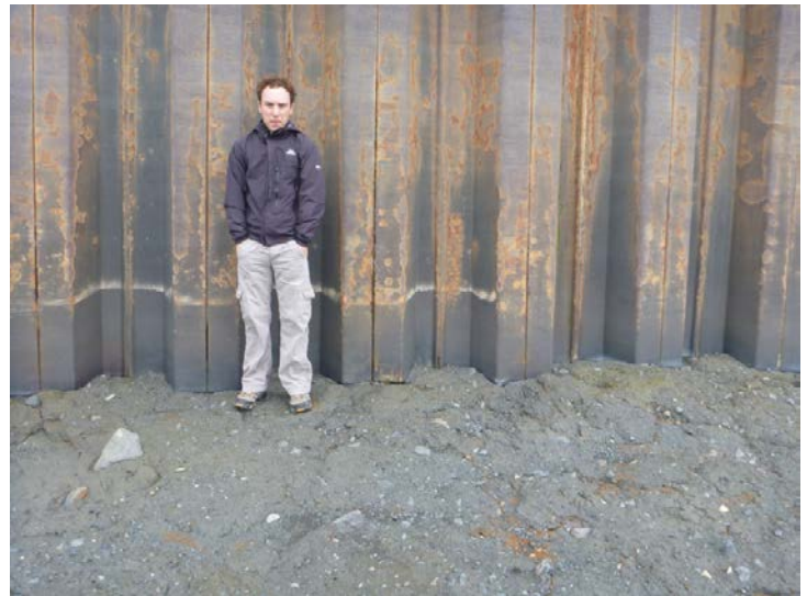
The newly-exposed bottom section of seawall illustrates rapid coastal erosion in Dillingham, AK.
