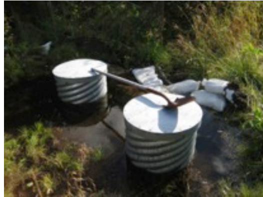
Figure 16. Perryville's source water infiltration gallery.
