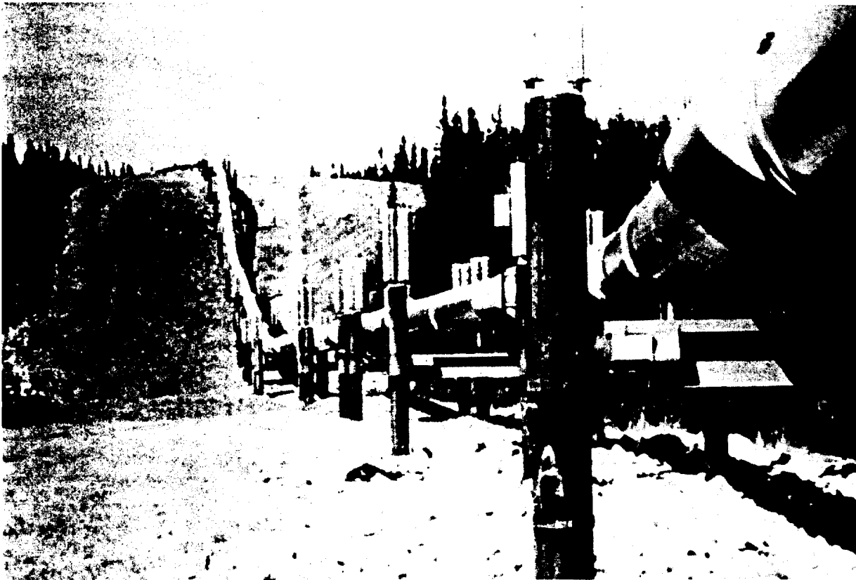
PLATE 5.2-4 Typical section of the Alyeska Pipeline in elevated mode. 'Cryoanchors' will be installed where necessary to prevent thawing of the permafrost in the discontinuous permafrost regions. (Courtesy: J. DenBeste, Aquatic Environments Limited).
