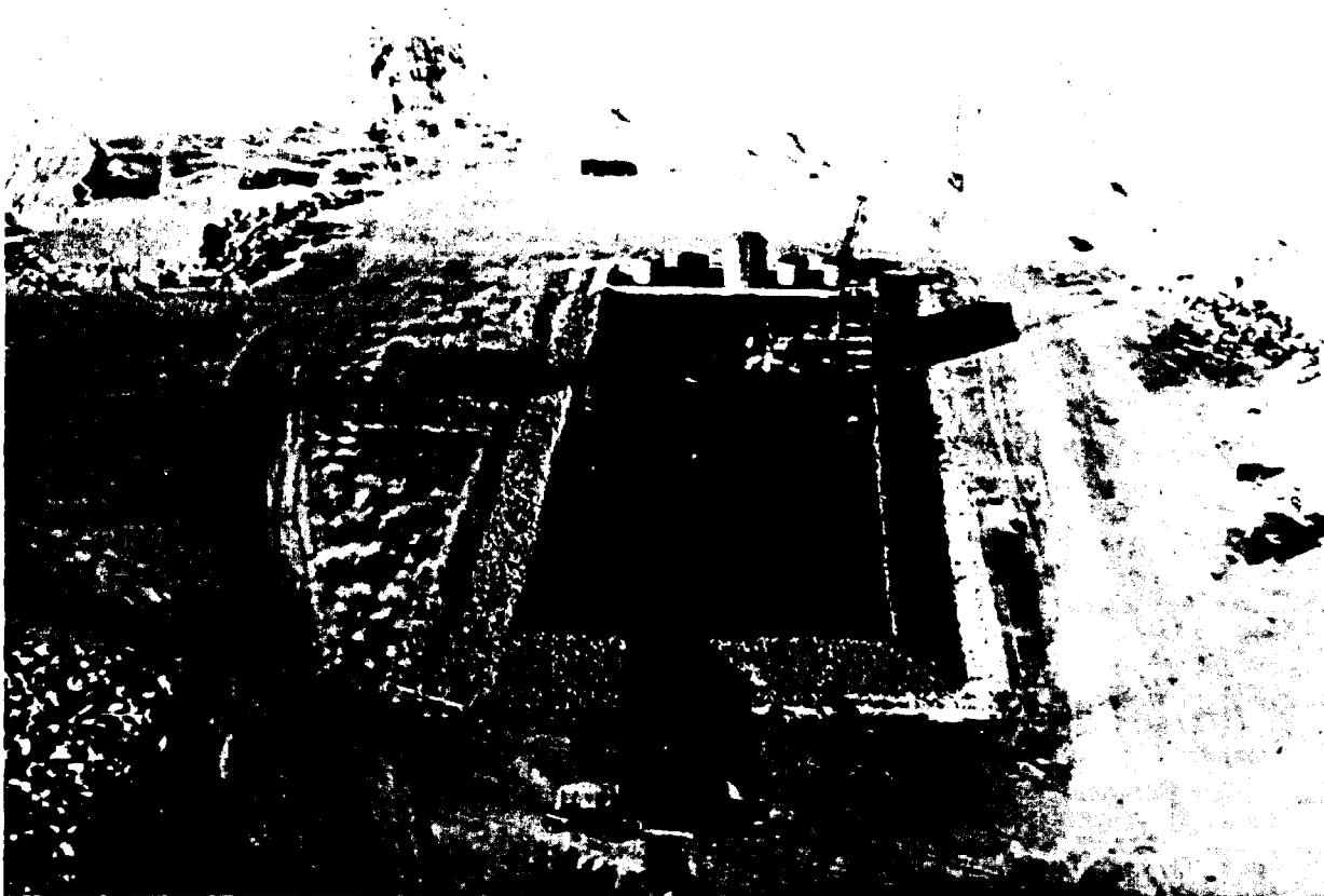
PLATE 3.6-4 In shallow waters of the Beaufort Sea well clusters will be located on production islands similar to this exploration island at Adgo.
