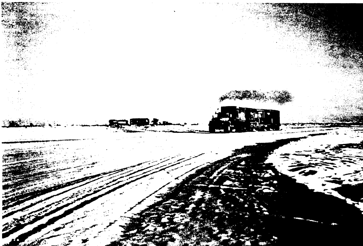
PLATE 3.6-2 Winter ice roads provide ready access to production or exploration locations, granular borrow, or other sites throughout the Mackenzie Delta and nearshore Beaufort Sea.
