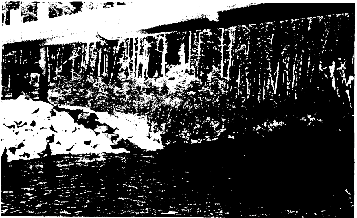
PLATE 5.2-3 An elevated section of the Alyeska Pipeline at a stream crossing. Note banks armoured with rip-rap. Installed in winter, these crossings have been shown to have little or no effect on aquatic resources. (Courtesy: J. DenBeste, Aquatic Environments Limited.)
